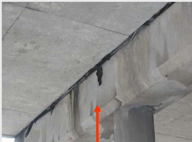
Asphaltic roofing felt or fiberboard bearing material
