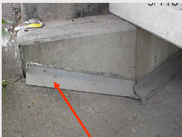
Mastic used to adhere flashing
